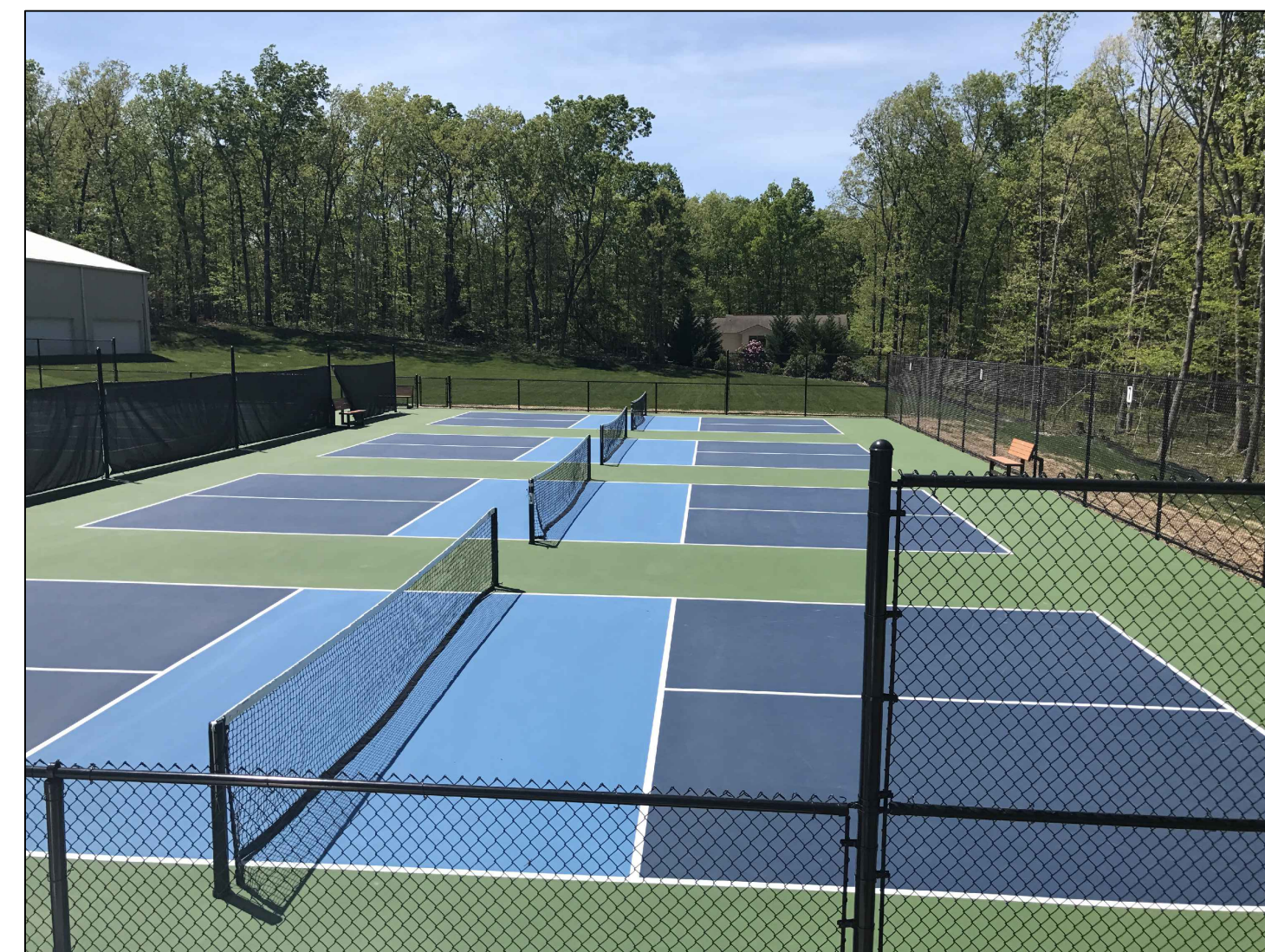
COURT COLORS CONTRACTOR TO PROVIDE MANUFACTURER SAMPLES TO ACHIEVE THIS COLOR COMBINATION.
